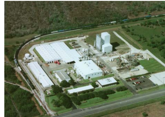
Catalyst plant in Houston, Texas
