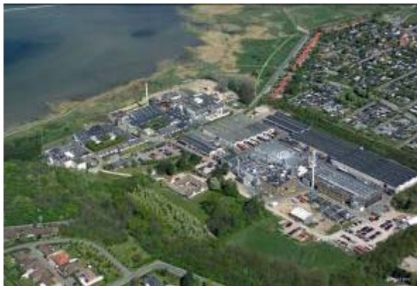
Catalyst plant in Frederikssund, DK
